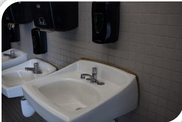
Antiquated facilities and fixtures
