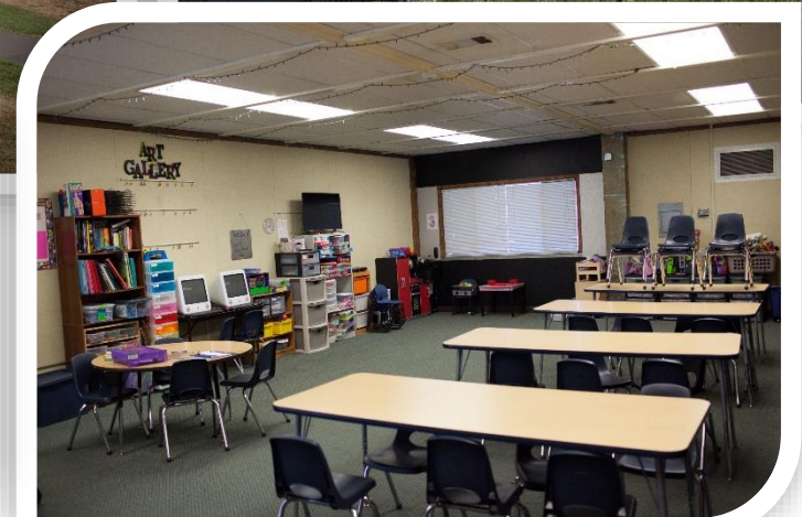
Deteriorating temporary portable classrooms need to be replaced
