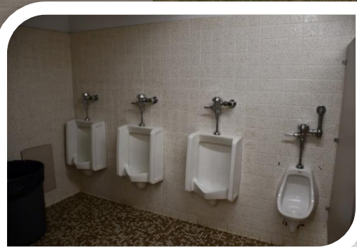
Renovated bathrooms needed
