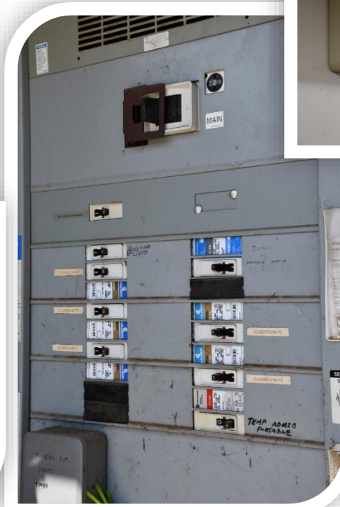
Outdated electrical systems
