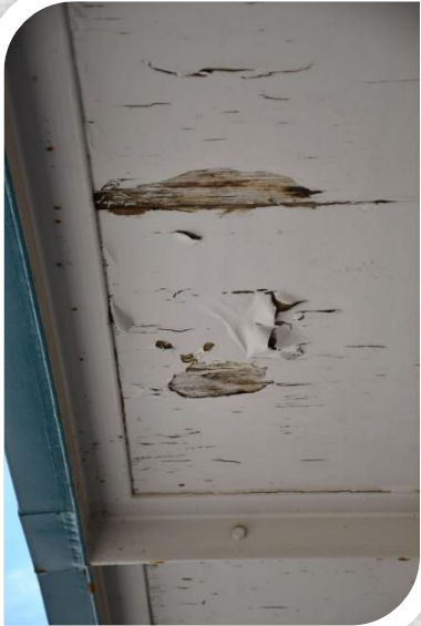
School facilities need repairs
